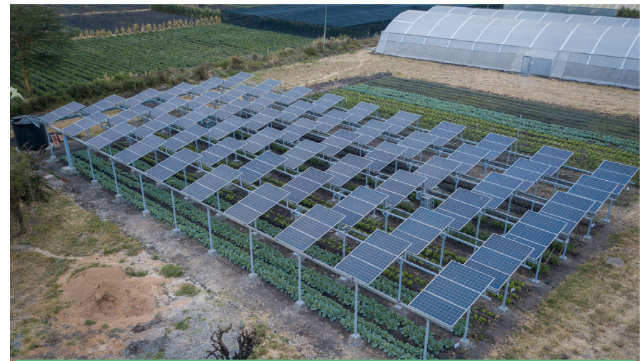
Figure 8: Smaller PV Modules 20
