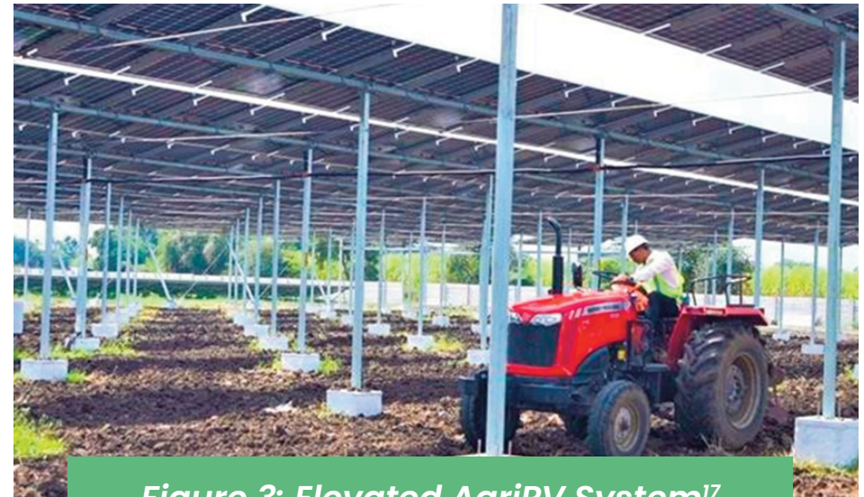
Figure 3: Elevated AgriPV System 17
